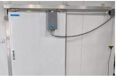
In addition to providing good insulation properties and enhanced waterproof seal, the **CL-1750-E** gives you the automation you need to improve your day-to-day operations. Over time, Norbec sliding doors have become a standard in the supermarket and food processing industry for their ease of operation, robustness and energy efficiency.
